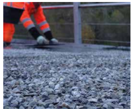
13 Splittstreuung in UHFB-Schlämme © Emch+Berger AG Bern
