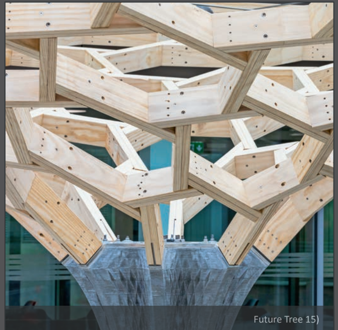
Cultivation and new construction Harder Kulm, Interlaken 5)
